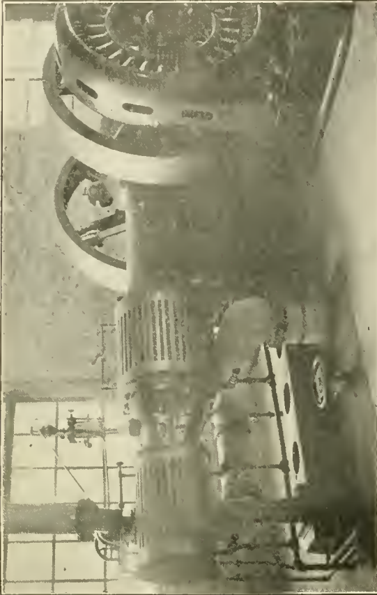
THE 10 X 16 X 14 TANDEM COMPOUND BALL ENGINE, WHICH DRIVES THE 60-KW. STATIONARY ARMATURE GENERAL ELECTRIC GENERATOR.
